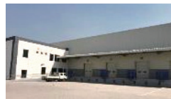
Dubai Warehouse the UAE
